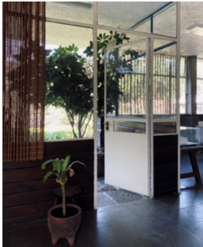
Fig. 23 Current view of the windows on the eastern terrace and the living room looking west, Agua 130, 2020. Photos: Martín L. Guzmán Elías and Thomas Hungerbühler.
