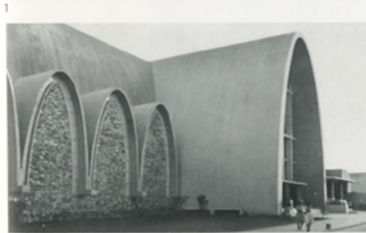
Church of Mary, Monterrey, 1947 Architect: Enrique de la Mora
