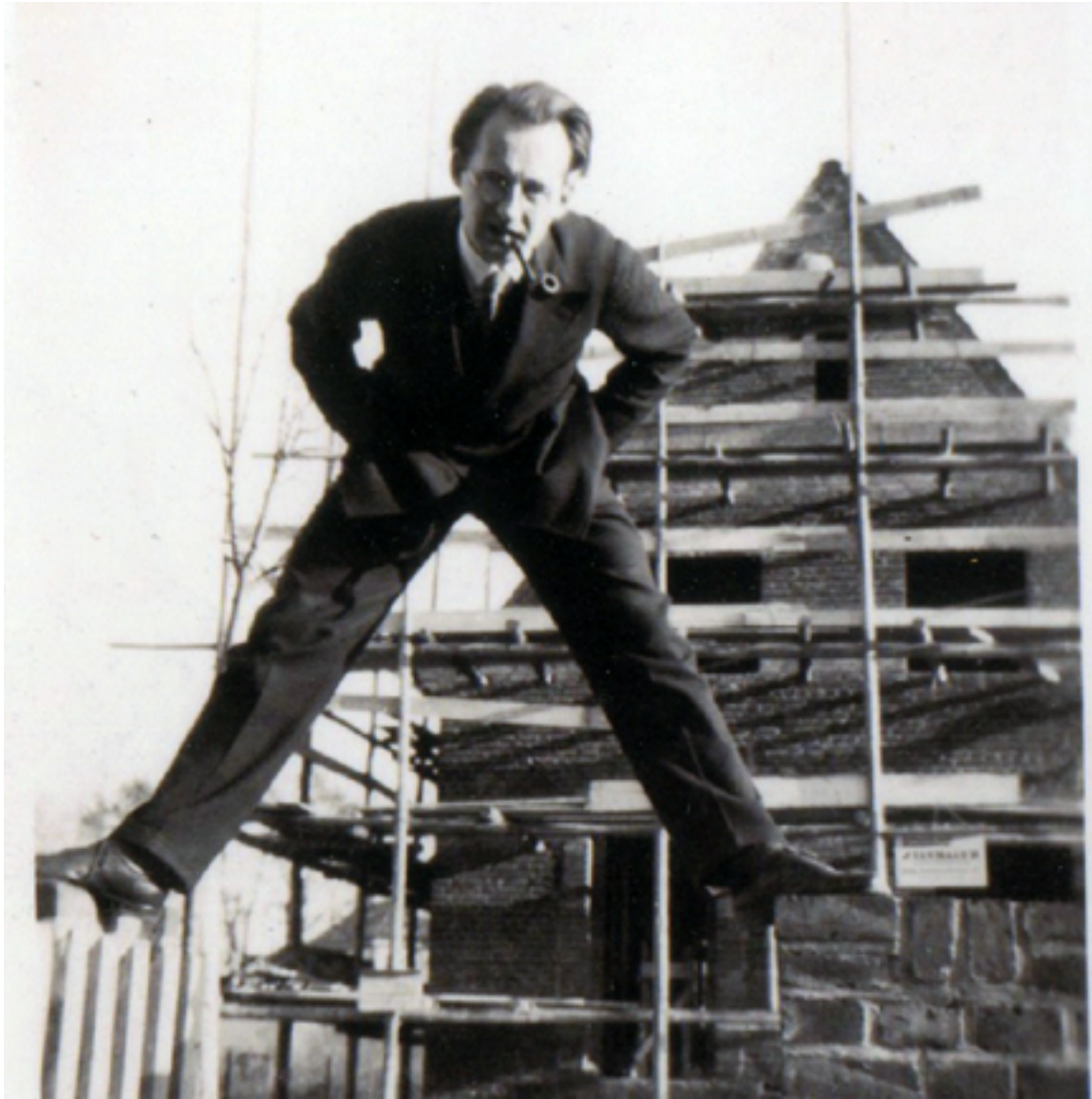
Cetto in Braunsberg, Germany, ironically simulating an old-fashioned roof, 1933, Bettina Cetto Archive.
